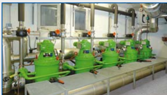
Fig. 3 river water filtration for cooling plant
