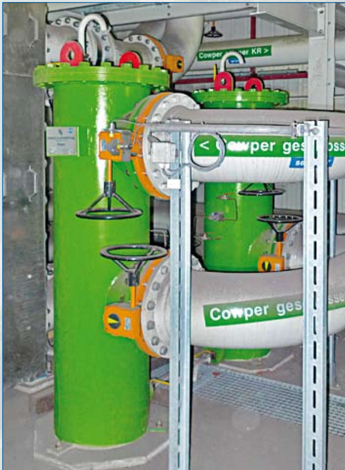
Fig. 2 Single Filter in welded steel design
