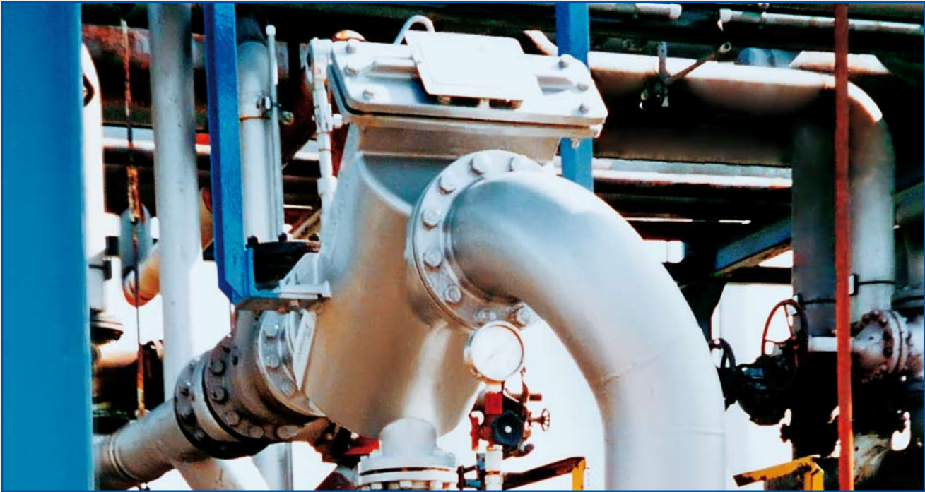
Fig. 10 oil filtration in a refinery
